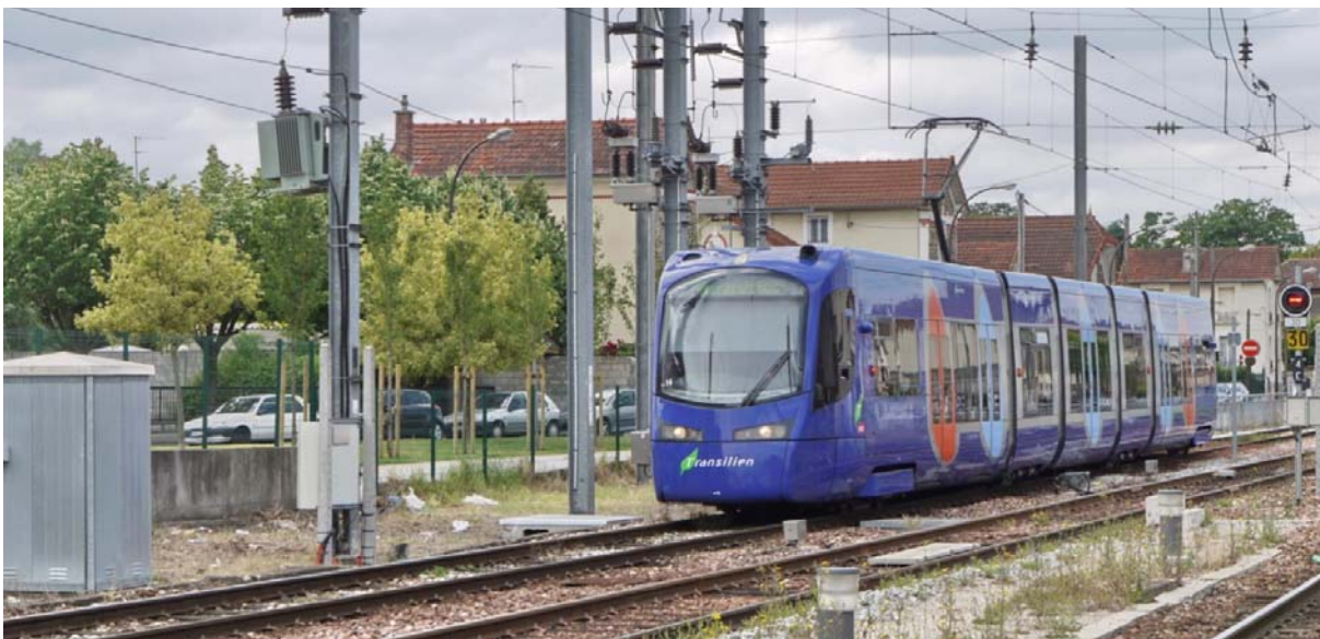
Figure 8. A tram-train on the Paris tram line T4 in June 2010. The Siemens-built Avanto S7 is composed of five units, with a total length of 36.5 meters.
