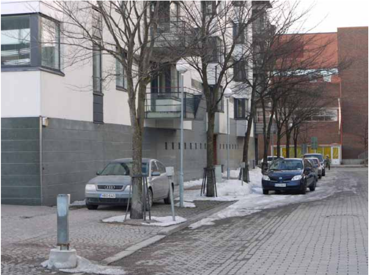
Figure 11. Dedicated curbside parking with heating poles in Ruoholahti at Kasuunikuja. The street is public street but the parking slots are private. While the poles are in row with the trees, there is no need to plough snow near the poles. This organization differs from the situation in the city centre by the dimensioning of the street width. There are no tree rows in the city and the lane width between parked cars may remain less than 3 meters.
